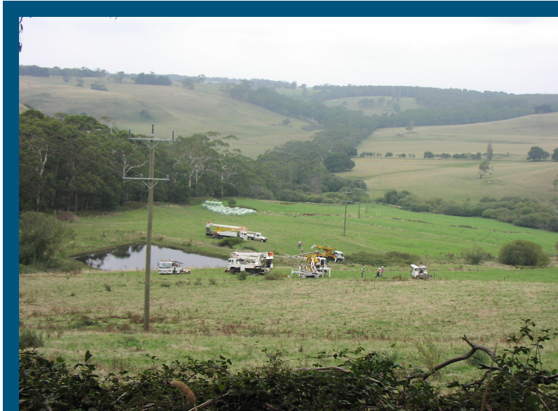
Powercor Line Crews preparing to stand Poles into Live 22kV conductors
