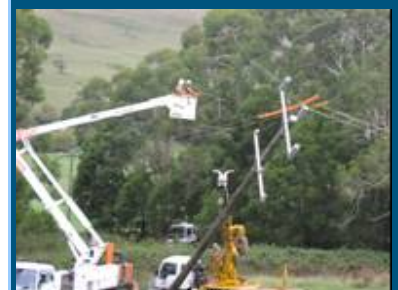
A Powercor Australia crew Stand a Pole into Live 22kV Conductors
